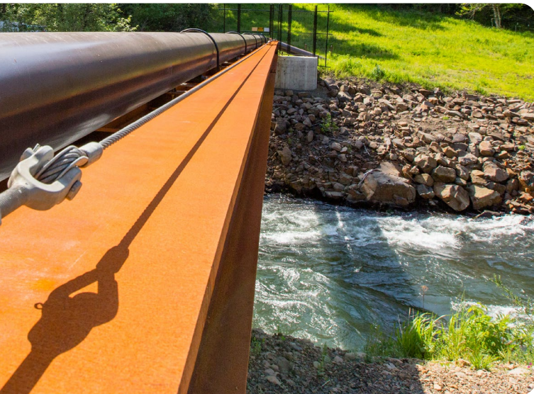
Northwest Pipeline in Hood River, Oregon.
