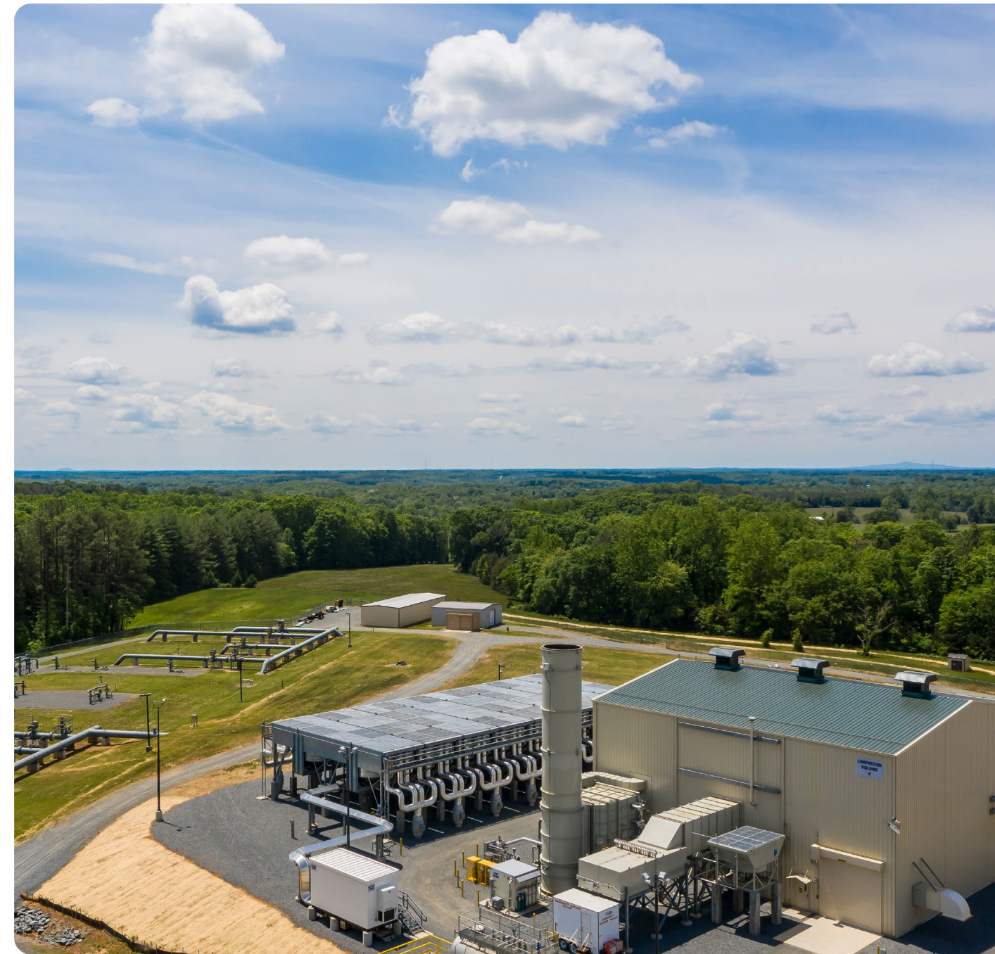
Transco Pipeline in Virginia.
