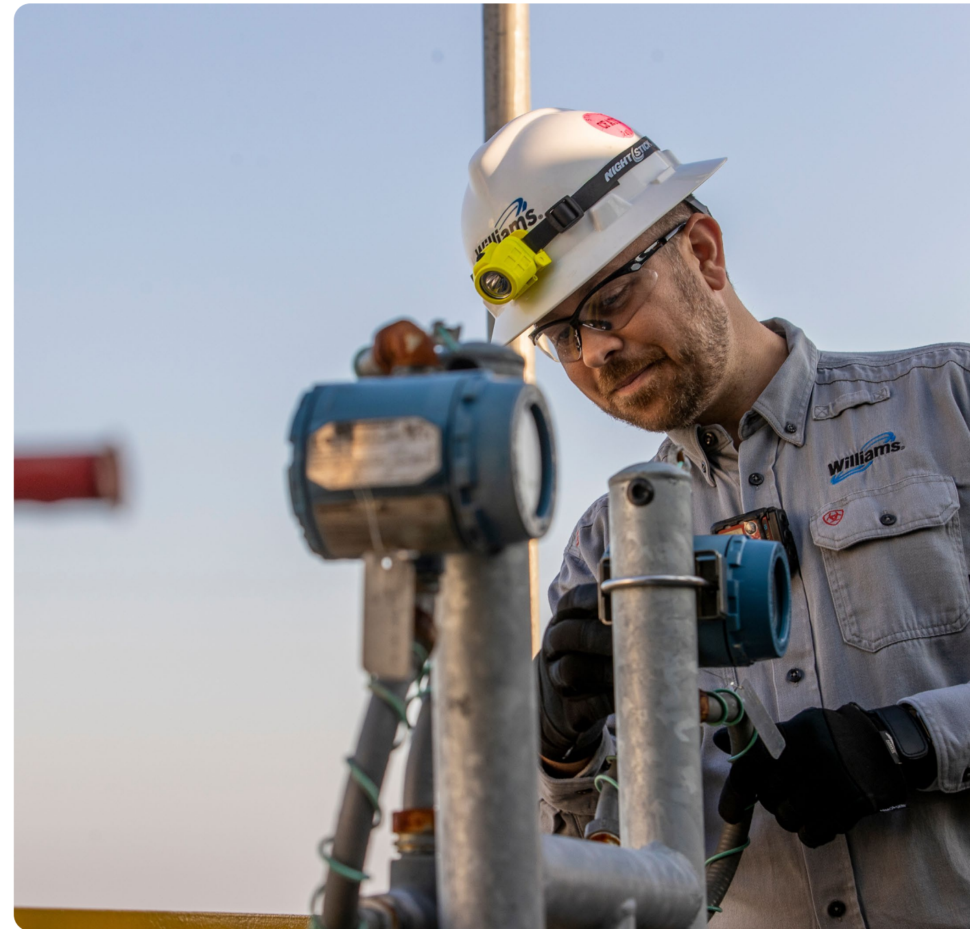
Nathan Carlson, WORK Experience Product Owner at the Transco Pipeline Station 240 in Carlstadt, New Jersey.
