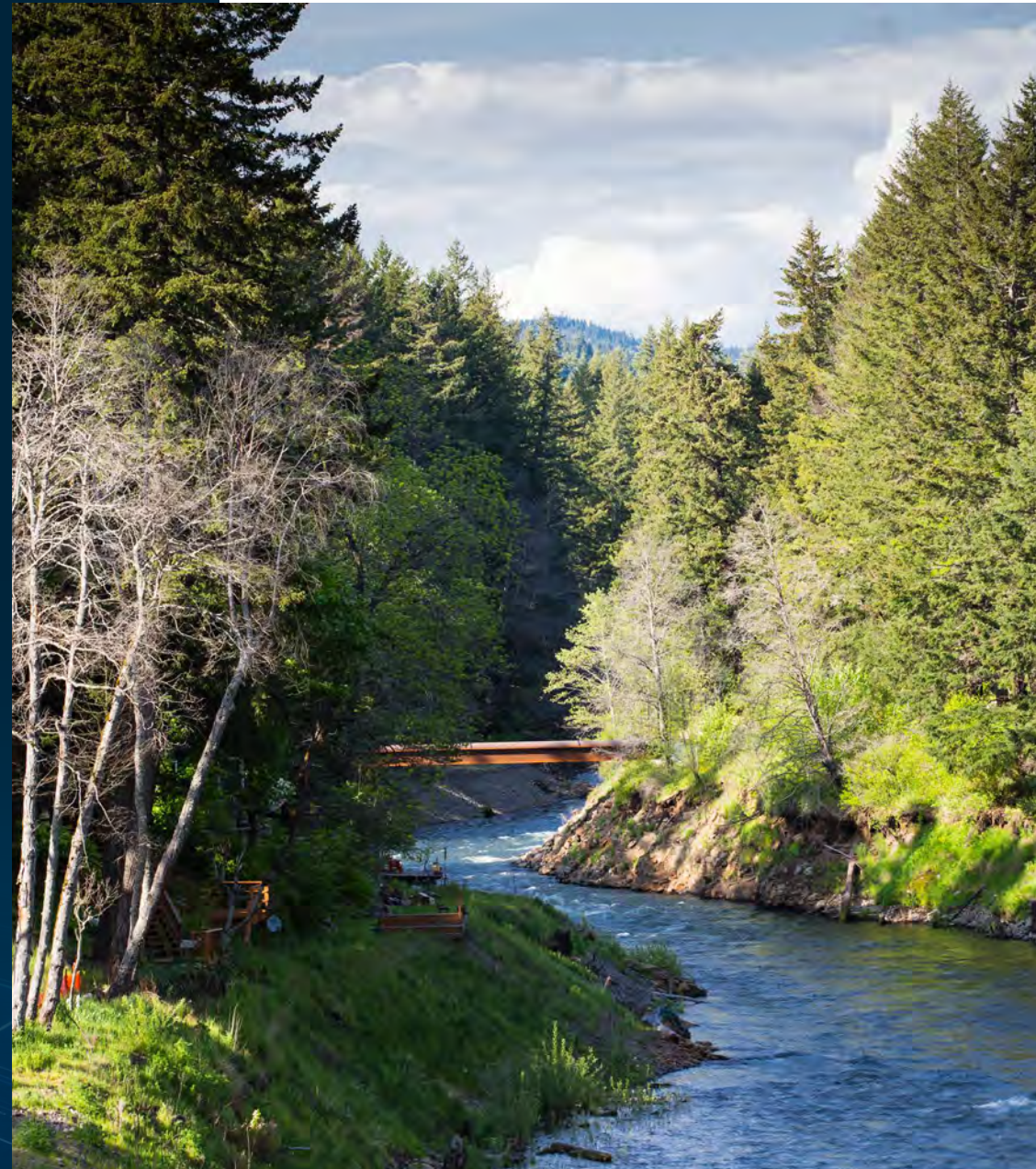
Northwest Pipeline over the White Salmon River near White Salmon, Washington.
